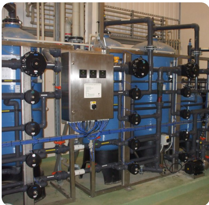
The installed Deioniser and Reverse Osmosis Plant as seen on site
