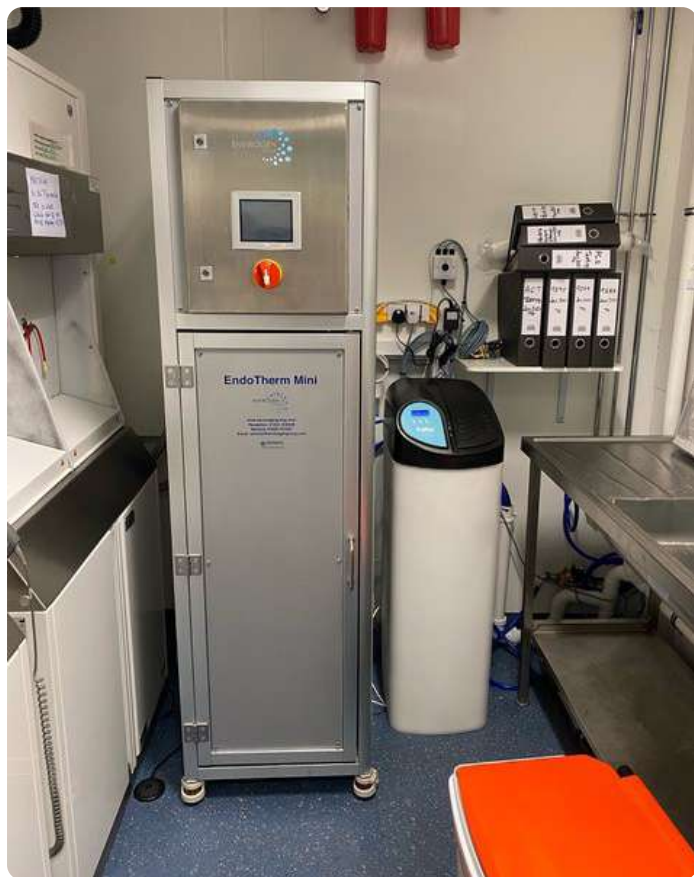
An Envirogen EndoTherm Mini reverse osmosis hire unit enabled the department to maintain service while the scheme was completed
