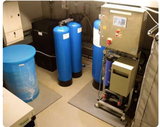
The Envirogen EndoTherm Duo Modular skid-mounted duplex RO system provides 100 percent resilience
