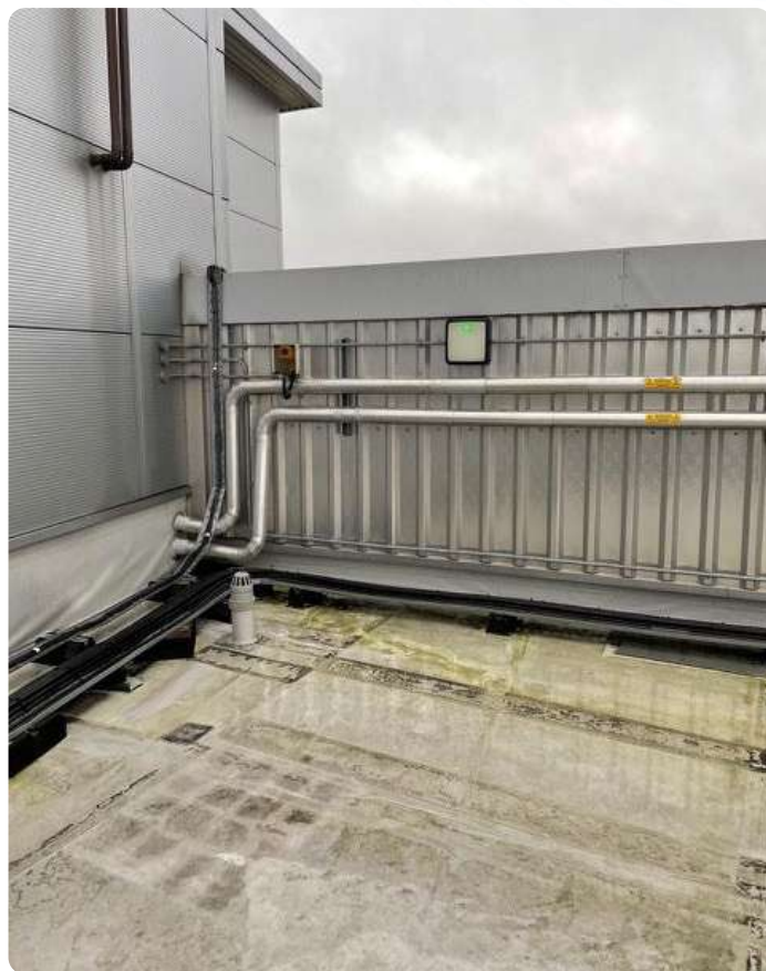
The extensive stainless steel ring main runs 180m from the plant room to the endoscope reprocessing unit
