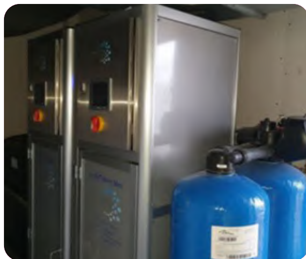
Duplex EndoTherm 500 Mini reverse osmosis system and ancillary pre-treatment equipment (water softener) inside a Vanguard modular mobile facility.
