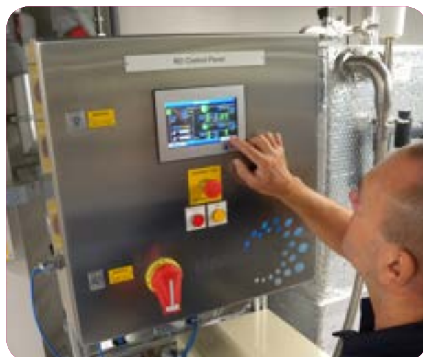
Stuart Macdonald, estates decontamination engineer, The Mid Yorkshire Hospitals NHS Trust, checks the RO system's control panel
