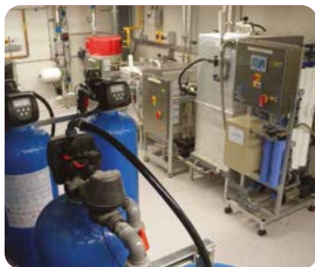
The Envirogen RO System at Pinderfields comprises three water softeners and two carbon vessels. The compact and flexible EndoTherm Duo Modular range can operate at elevated temperatures. This makes it ideal for all SSD applications - including disinfectors and sterilisers etc.
