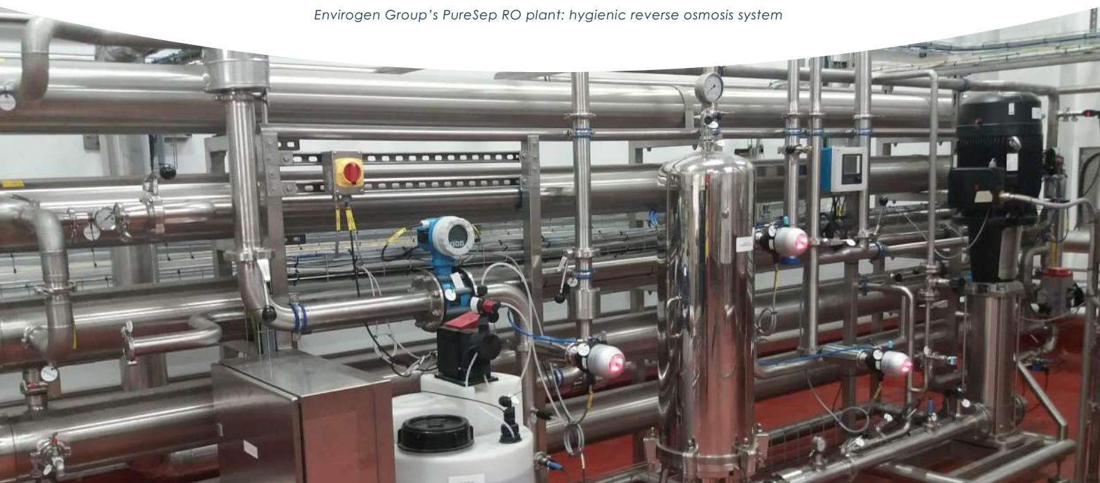
Envirogen Group's PureSep RO plant: hygienic reverse osmosis system
