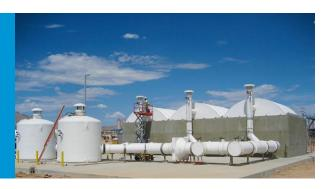
Envirogen Built-in-Place Biofilters are custom designed solutions for mid- to high-air flow VOC and odor control applications. These systems are employed in point source or centralized emissions control applications, for air flows ranging from 1,000 to well over 100,000 cfm. Installations are based on standardized system components and multibay designs to lower installed costs, increase flexibility of design and allow for expansion as plant needs change.
