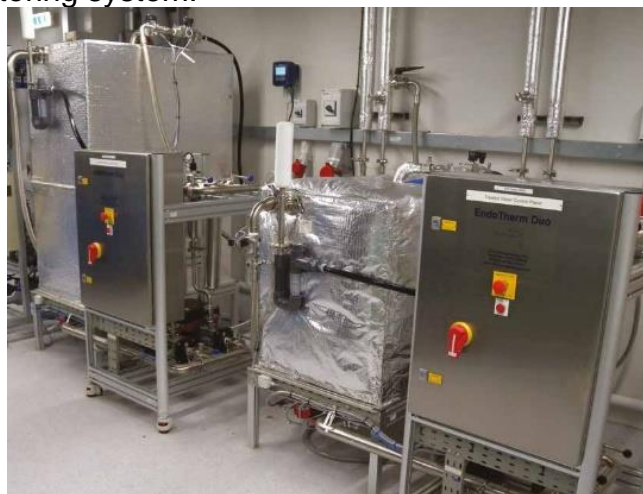
An Envirogen Group EndoTherm Duo Modular reverse osmosis system.
