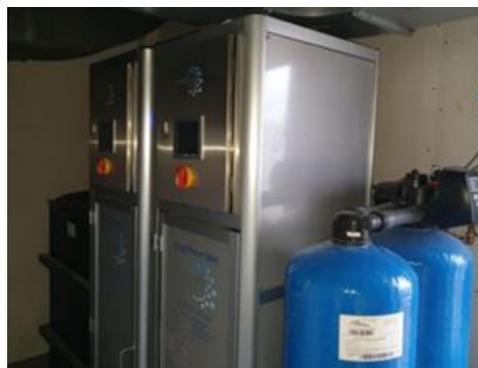
*Duplex EndoTherm 500 Mini reverse osmosis system and ancillary pre-treatment equipment (water softener) inside a Vanguard modular mobile facility.*
