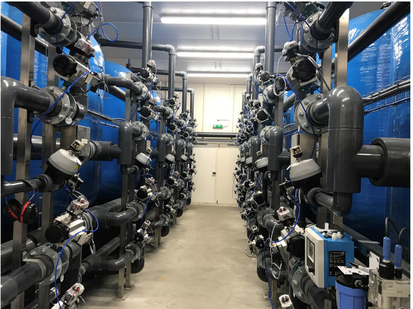
Activated carbon filters remove chlorine, odour and taste taints
