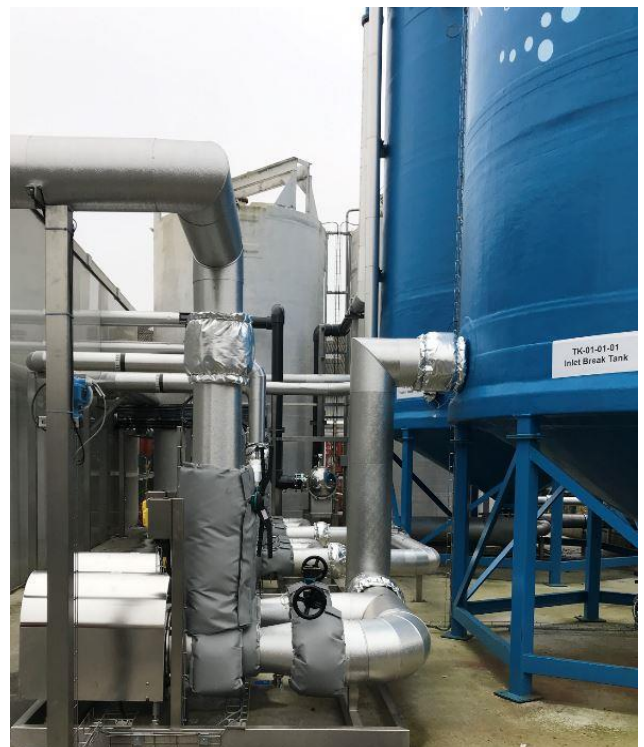
Chlorine dosing in the inlet break tank oxidises trace metals
