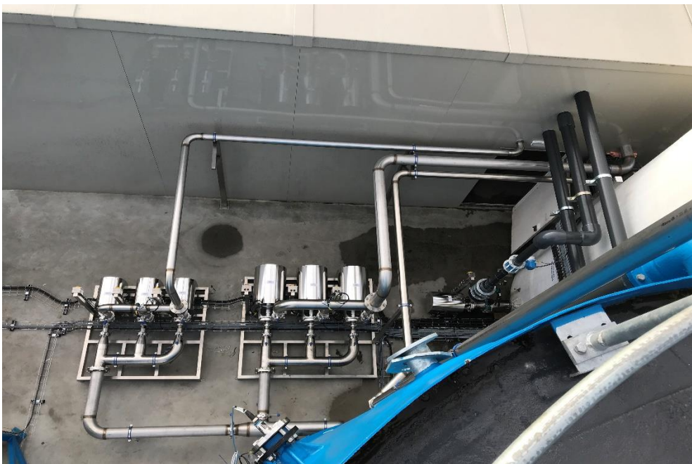
Aerial photograph taken during construction of borehole water treatment plant, Selby
