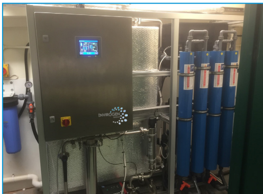
Compact Endotherm Duo: A complete water purification system with duplex RO units in a single frame.
