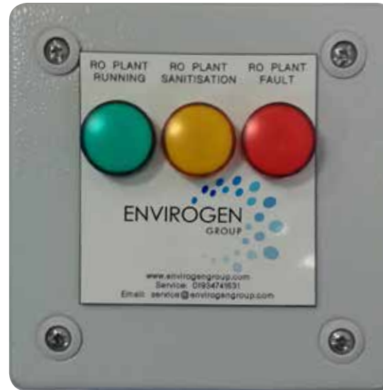
Remote wall-mounted alarm indicator
