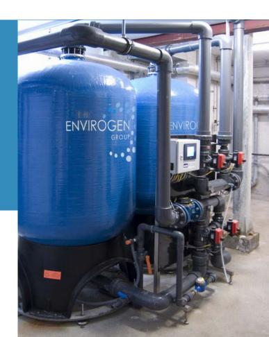
The combined effect of counter-current regeneration and rinse water monitoring is unique to the EcoSave system ensuring softened water quality of less than 1ppm total hardness, whilst consuming much lower quantities of salt when compared to traditional systems.
