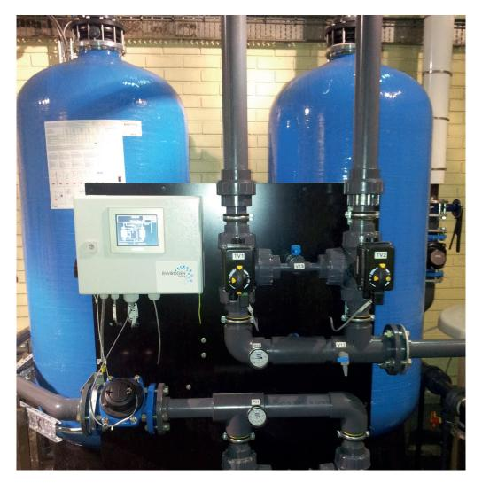
'The new system is fully automated and controlled through a HMI and PLC and 24-hour operation is ensured by having a duplex structure. One vessel is processing whilst the other is regenerating or in standby.'
